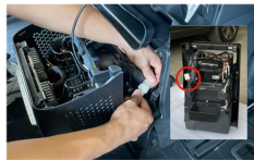
27.再把冰箱电源线与预埋取电线对接
