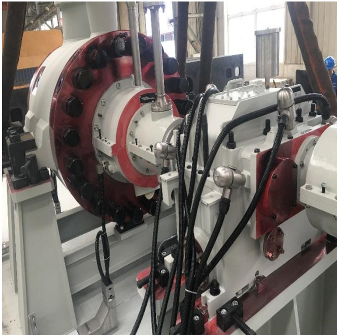
17. Painting Inspection of C2+ Regeneration Gas Compressor of product no ***)
